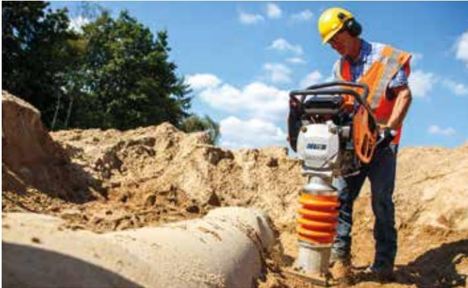
The new range of Hitachi compaction equipment shares the same qualities as Hitachi excavators and wheel loaders, such as reliability and durability. The ZV-R vibratory rammers are ideal for creating foundations and trenches in soil or sand. The ZV-PR reversible vibratory plate compactors are suitable for earthwork, road construction, landscape gardening and sewer-line construction. The TMR65KDS walk-behind roller is suitable for small compaction jobs incorporating paths, tarmac and sand.
